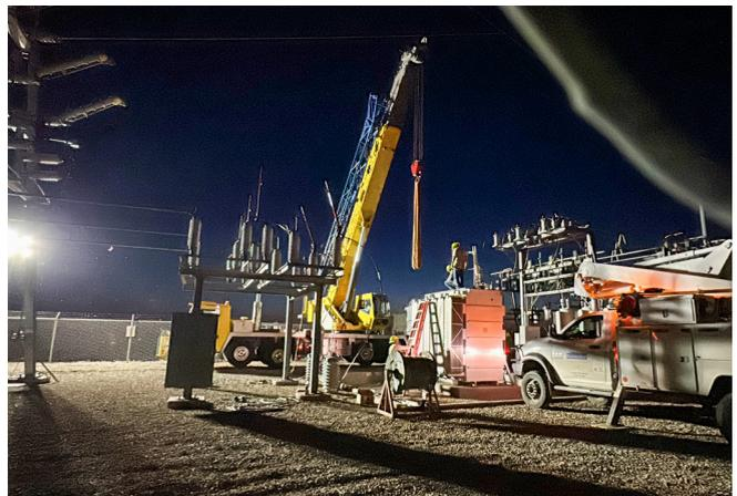
Out with the old, in with the new! Rolling Hills linemen use a crane to remove the damaged transformer and replace it with the new one.
