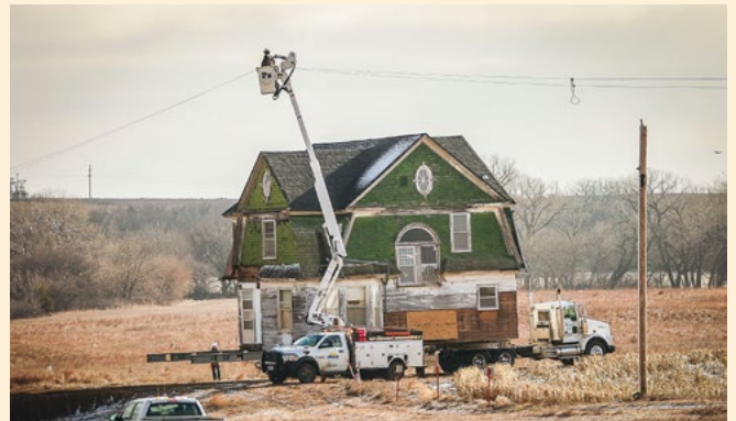
RHEC crew assisting with raising power lines for the house move.
