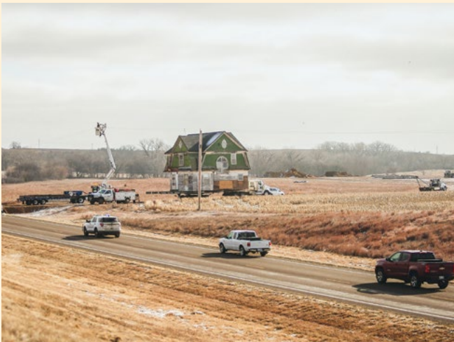
RHEC crew assisting with raising power lines for the house move.
